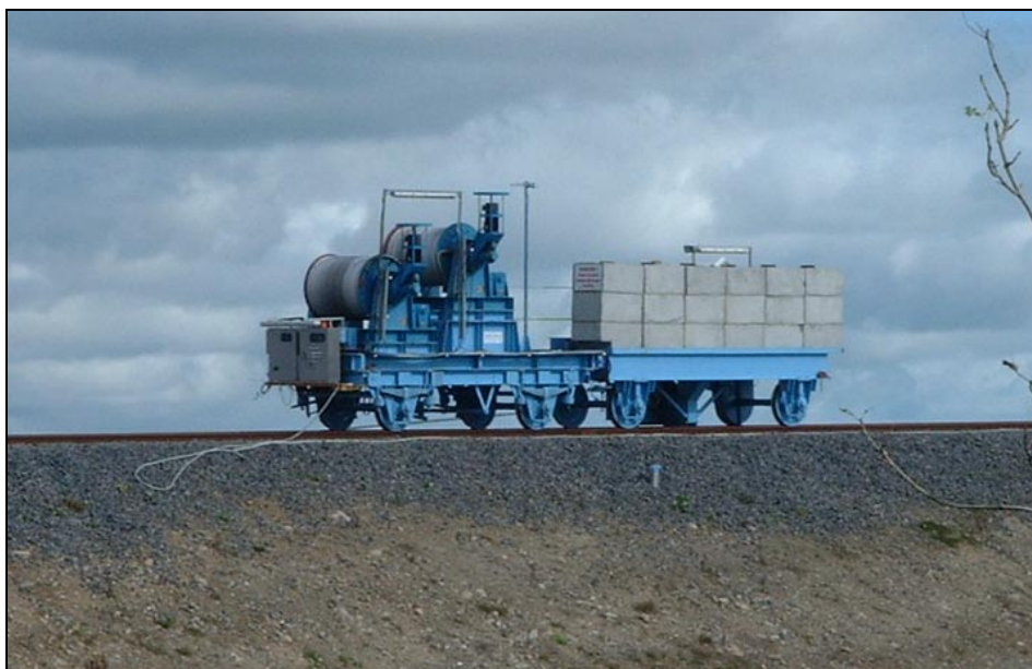
Figure 3.30: Electrically driven winch controlling the tailings distribution pipeline at the Lisheen TMF
