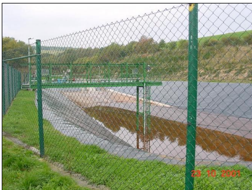
Figure 3.70: Water retention basin of German potash mine
