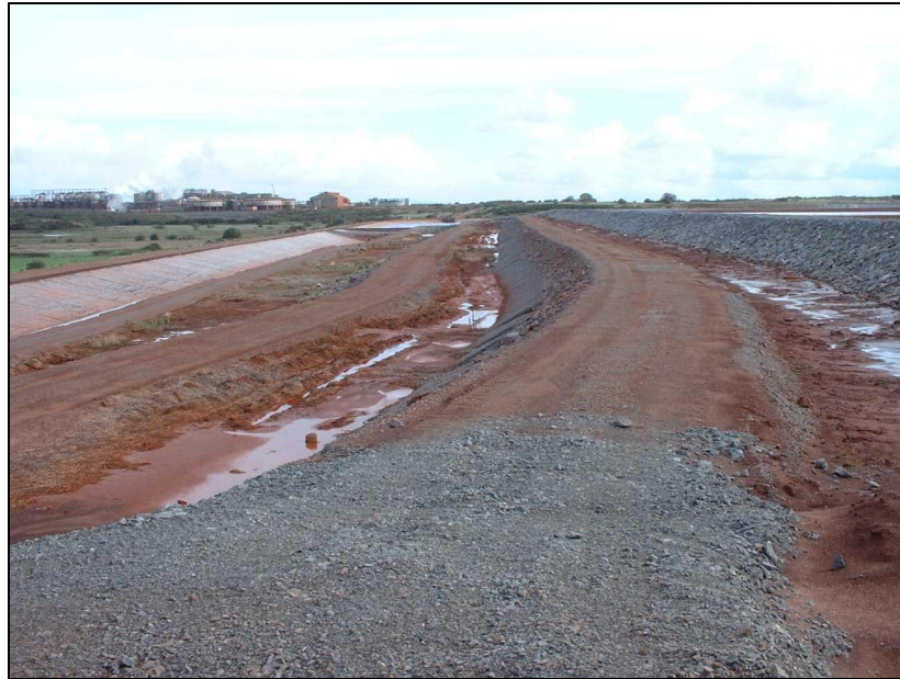
Figure 2.19: Dams raised using the upstream method at the Aughinish site
