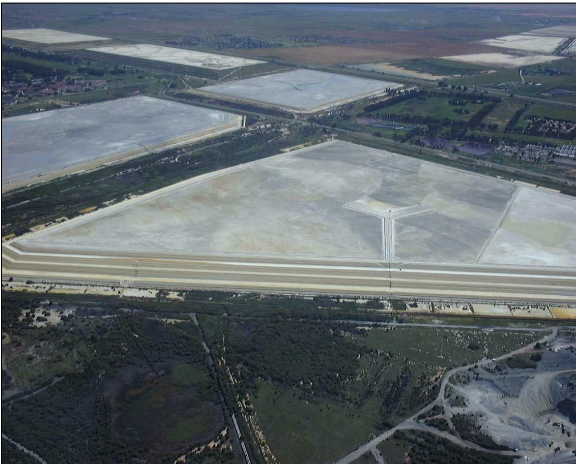
Figure 2.11: Tailings pond on flat land (Courtesy of AngloGold, South African Division)
